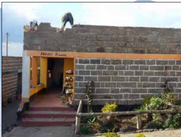
Renovation work on the roof of the camp
