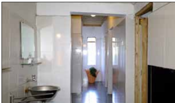
The new shower and bath room is now done
